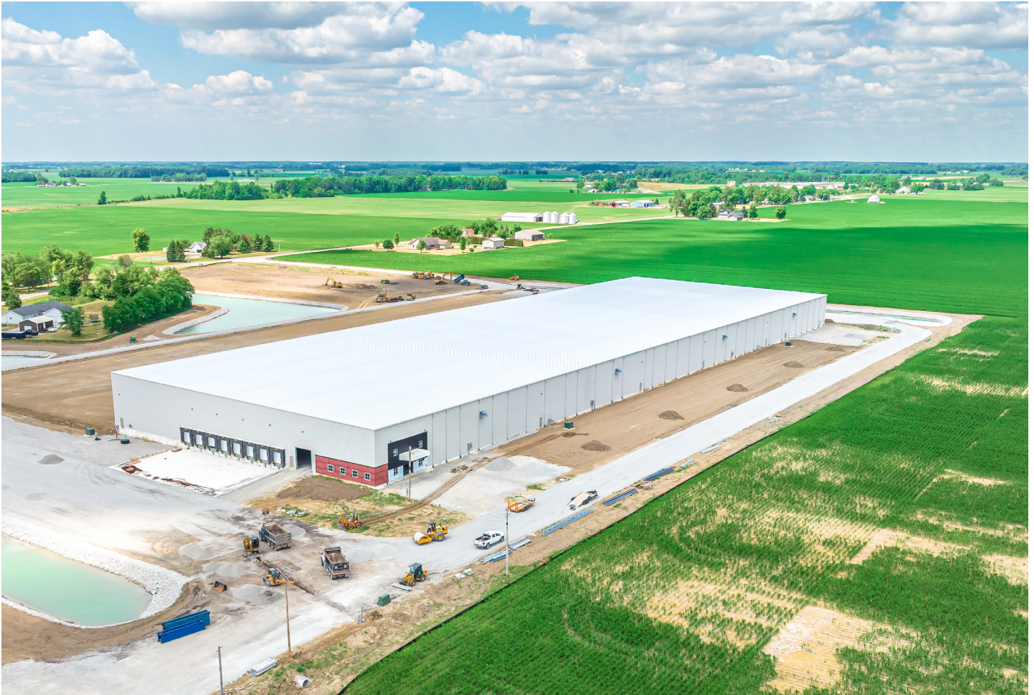
Spec Building, 859 Adams Street, Bluffton
