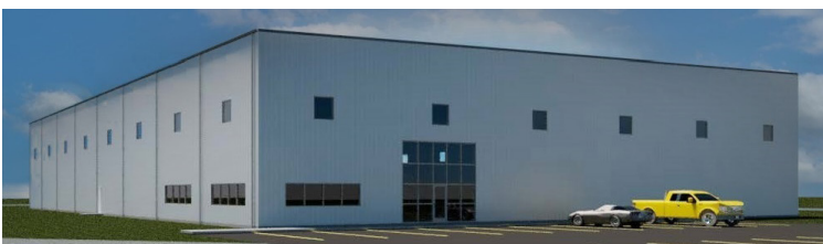
Spec Building, 435 Industrial Parkway, Ossian
